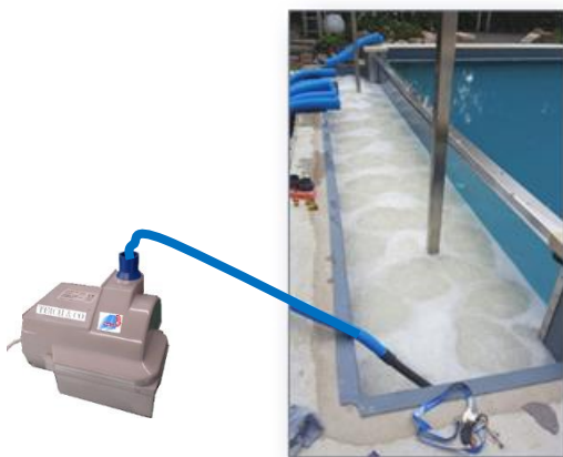
backflushing using the bubble pump
